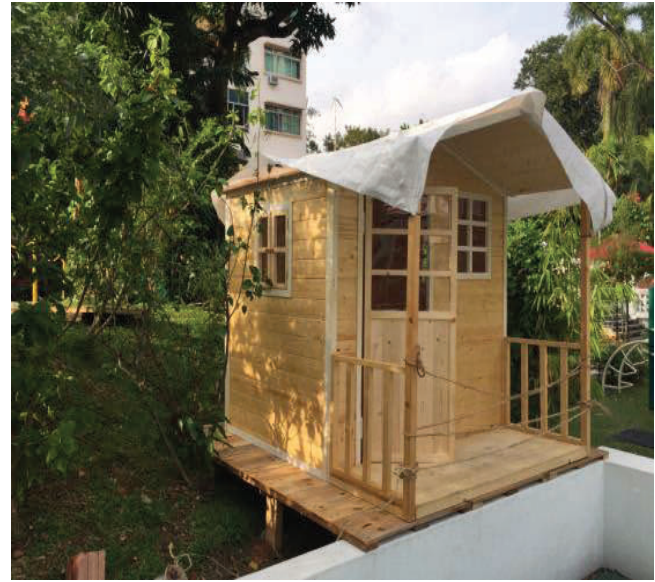
Photo 25: The completed playhouse
